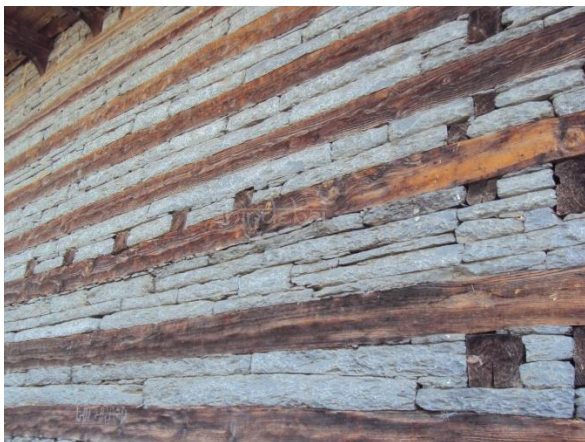
Fig. 1. Image showing Kathkuni construction technique- Jana, Himachal Pradesh
